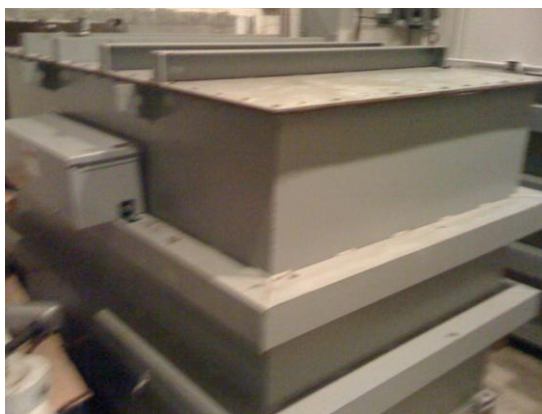
Figure 1. One of the two SF 6 HV-Platform Isolation transformers made by the Hammond Manufacturing Co. They can be operated in air up to at least 60 kV and with SF-6 up to 300 kV.
